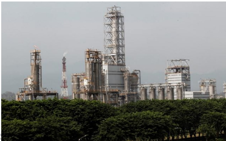
Existing PE plant in Cilegon with capacity 336 KTA where 1 train is UNIPOL PE Technology 200 KTA and another train 136 KTA is SDK
